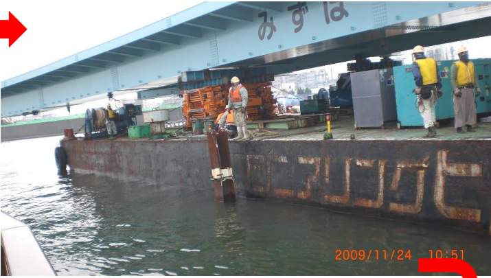
11/24 10:51架設場所の係留杭に接岸中
